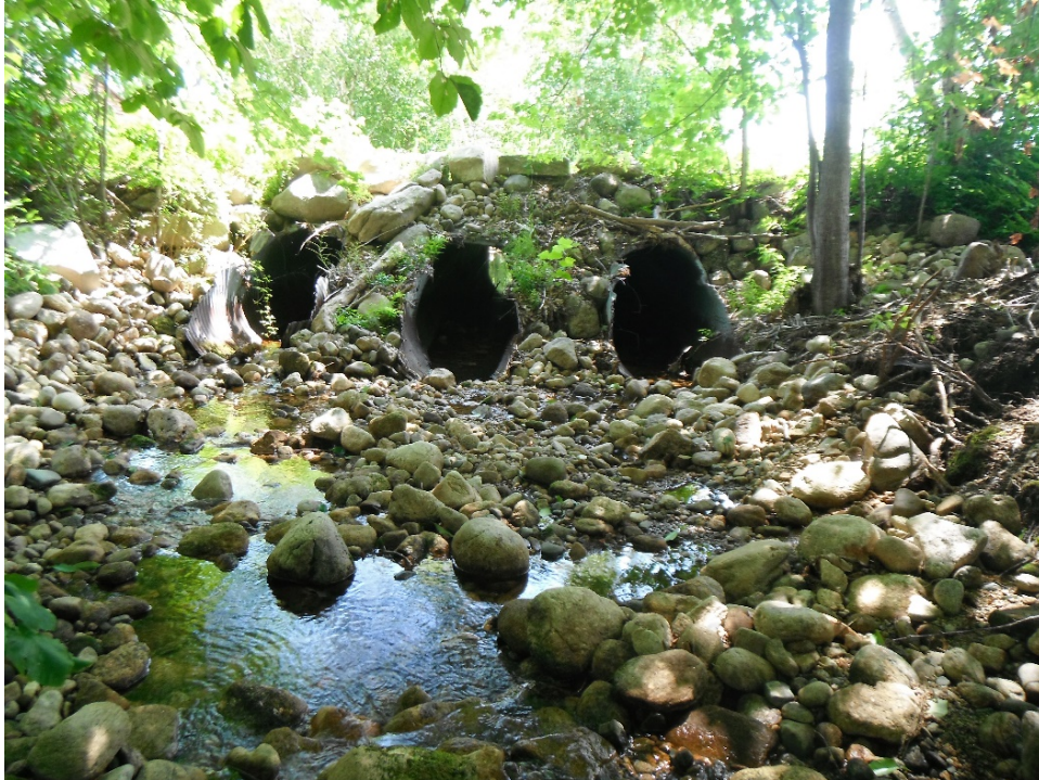
Photo 8. Three barrel culverts under Adams Road.
